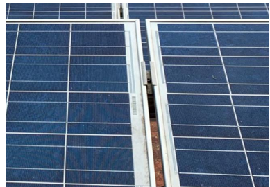
Fig. 2: Gap between the solar modules [1]
